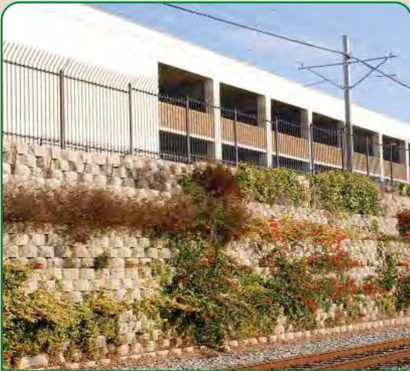
MTDB Laurel Street Crossing • San Diego, CA
